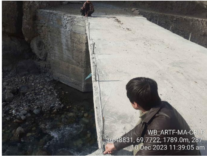
Figure 6: CRLP Rectified Critical Deviations: Guardrails on both sides of the bridge were not installed.
