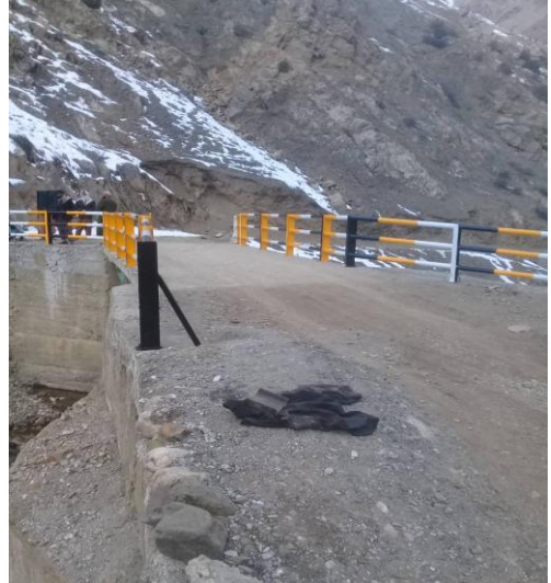
Figure 6: CRLP Rectified Critical Deviations: Guardrails on both sides of the bridge were not installed.
