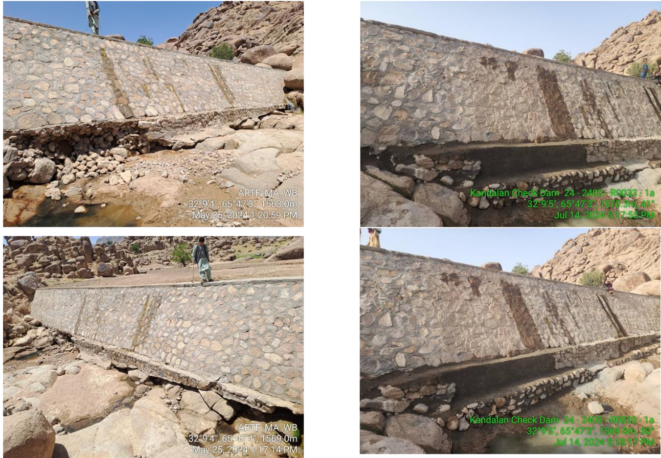
Figure 8: CRLP Rectified Major Deviations: Check dam foundation had been washed and scoured.
