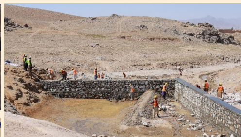
Construction of a Check Dam to Store Irrigation Water in Jaghatu District, Wardak Province
